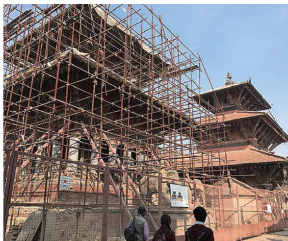
Figure 2. Damaged temples in Patan Durbar Square (November 14th, 2017 photographed by the author)
